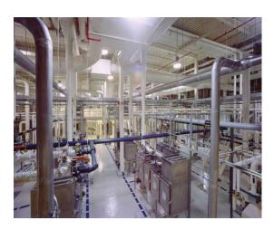
Smith Carter Architects requires contractors to produce detailed construction coordination drawings for all high containment facilities. The drawings are considerably more detailed than normally required and indicate where piping conduit and duct work will run to accommodate things like light fixtures, air distribution systems, sprinkler systems and electrical systems. (*Image courtesy of Smith Carter Architects.*)
